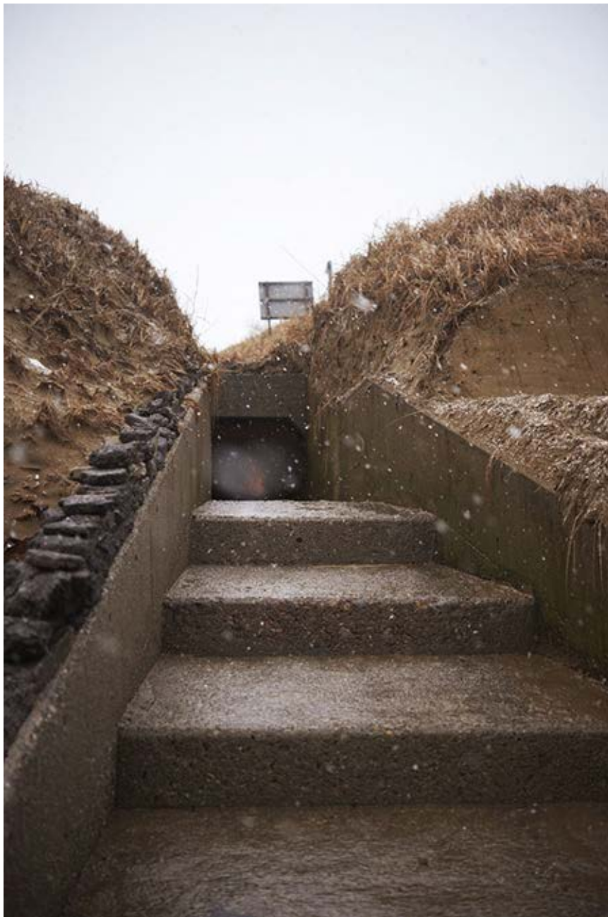
Still Image from ROAD CUT THROUGH A HILL
